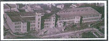
The original three-story main mill building was constructed in 1896, and is built of brick which was probably made on site. Windows are arched, typical in industrial buildings, and are all in filled with brick. Decorative brick
