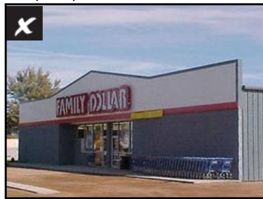
Plain Concrete Block and Metal Facade
