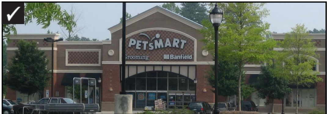
Façade with Recesses and Projections
