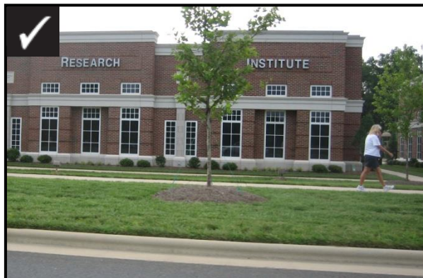
Parapet with Decorate Cap and Varied Roof Line
